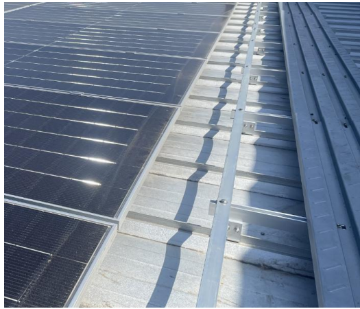
Fig.5 The roof is made of aluminum alloy
