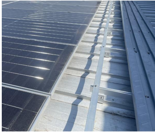
Fig.5 The roof is made of aluminum alloy
